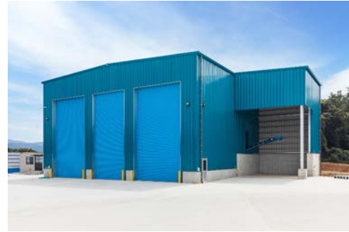
工場新築工事
